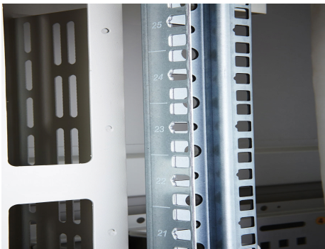
19" profiles marked with U height position
