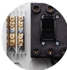
Example of internal 3-pole switch
